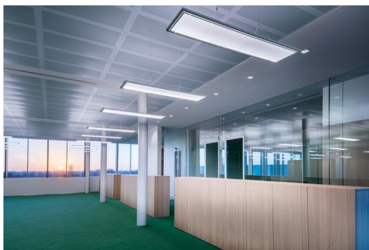
Figure 5: Office lighting with high-quality luminaires with sophisticated design. In case one luminaire fails and cannot be replaced or repaired (e.g. because components with that state of technology are not available anymore), all luminaires will be replaced.
